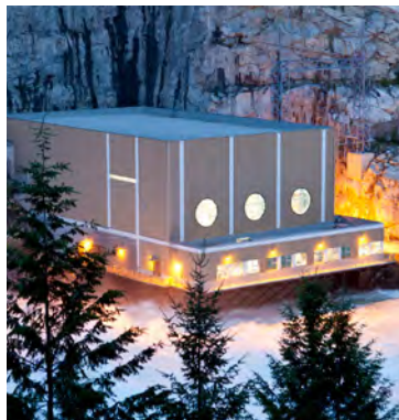
Brilliant Expansion Generating Station
