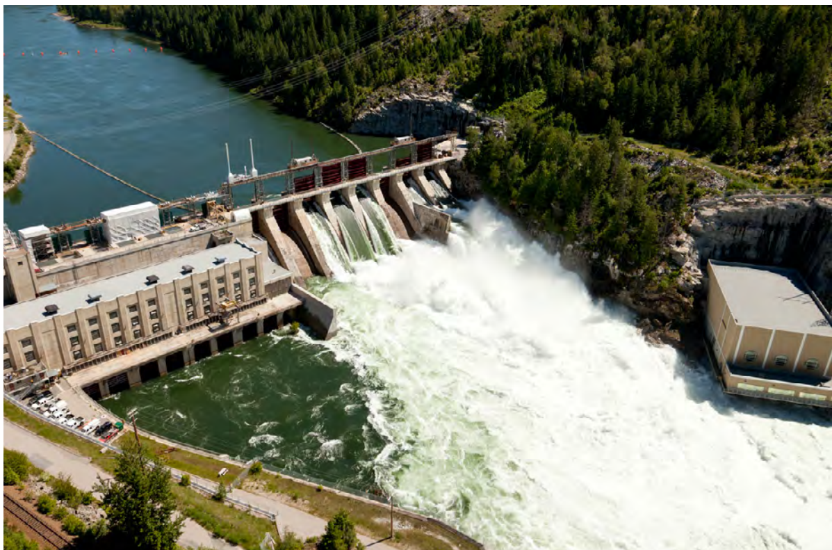
Aerial view of the Brilliant Dam and Generating Station and the Brilliant Expansion Generating Station
