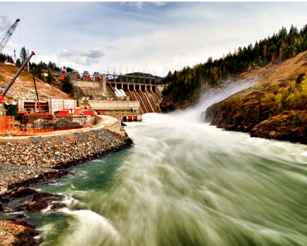
Construction of the Waneta Expansion Project
