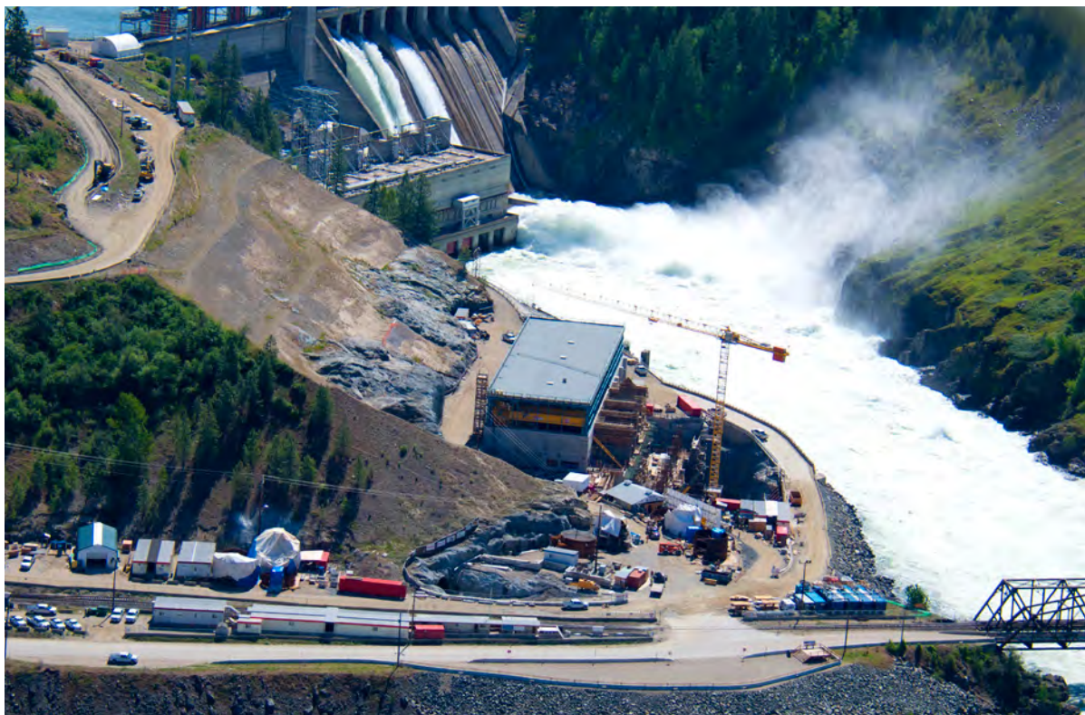
Aerial view of the new Waneta Expansion Project powerhouse
