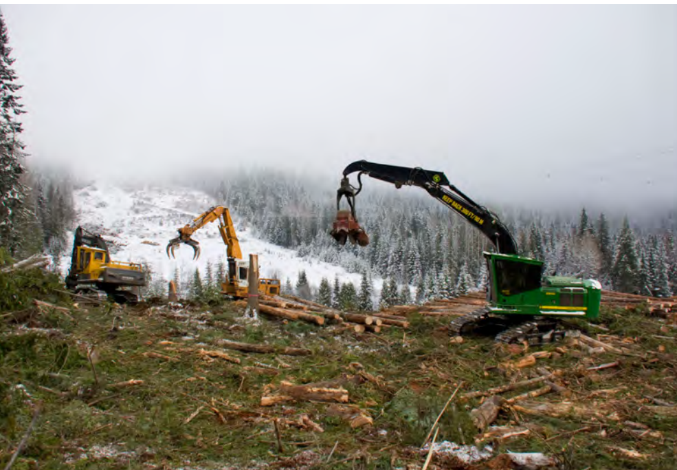
Logging and clearing work for the Waneta Expansion Project transmission line
