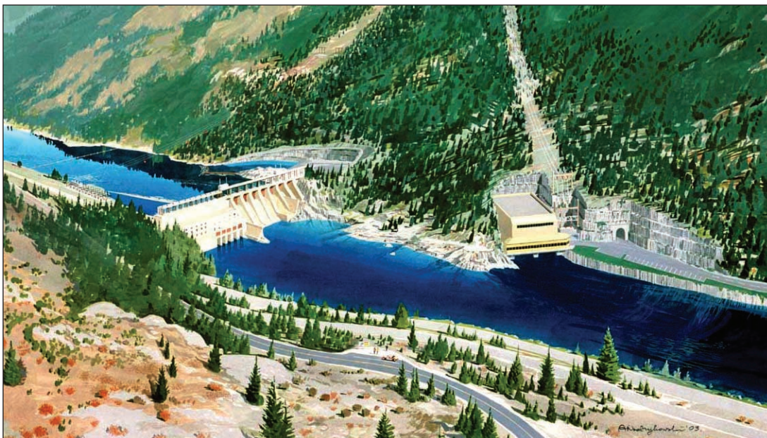
Artist's rendition of Brilliant dam and Brilliant Expansion (under construction)
