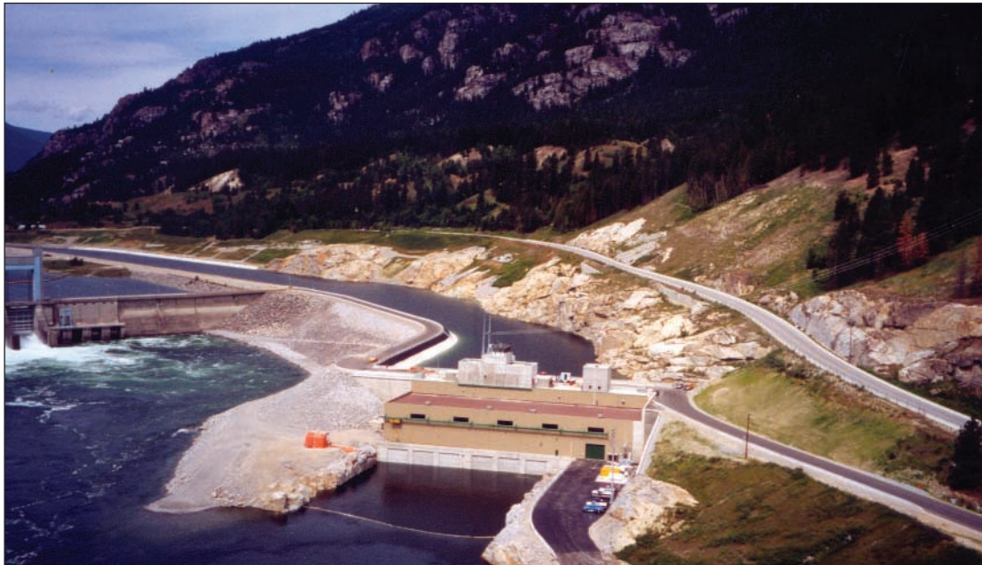
Arrow Lakes Generating Station
