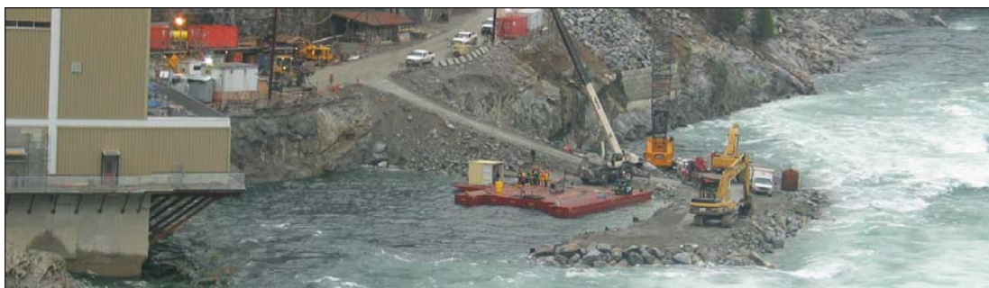
Removing berm at Brilliant Expansion
