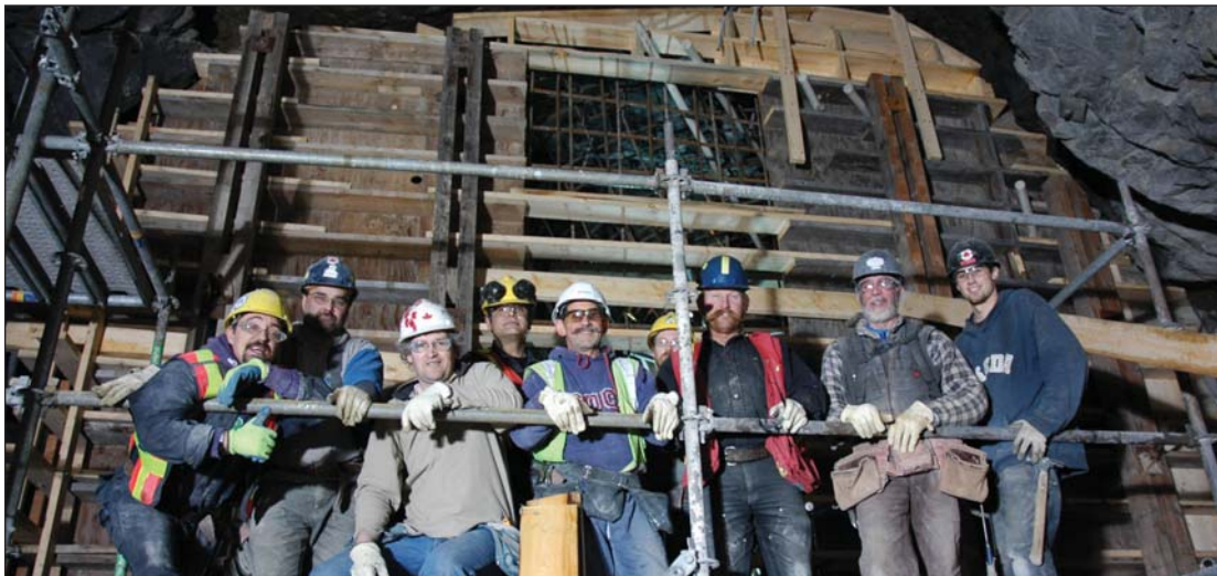
Adit plug formwork crew at Brilliant Expansion
