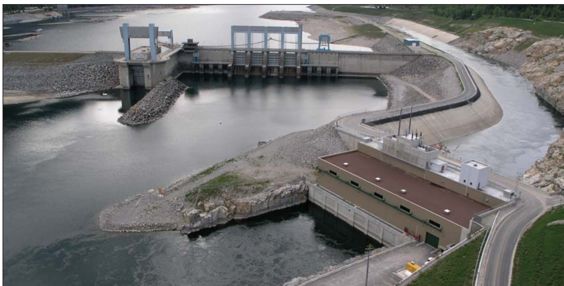
Arrow Lakes Generating Station located at the Keenleyside Dam on the Columbia River
