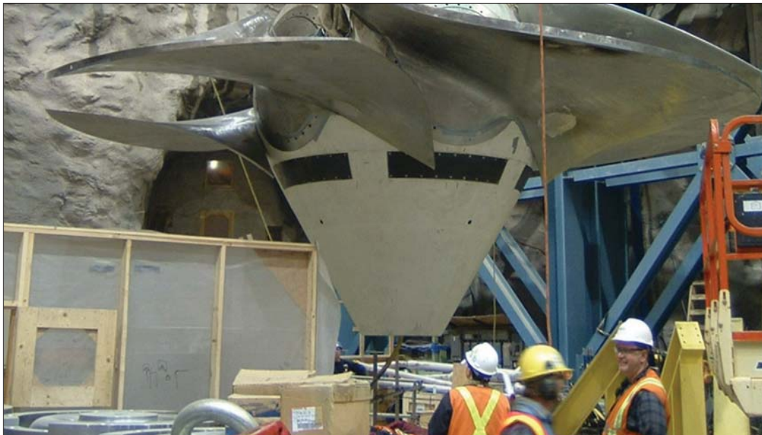
Crew installing turbine runner at Brilliant Expansion
