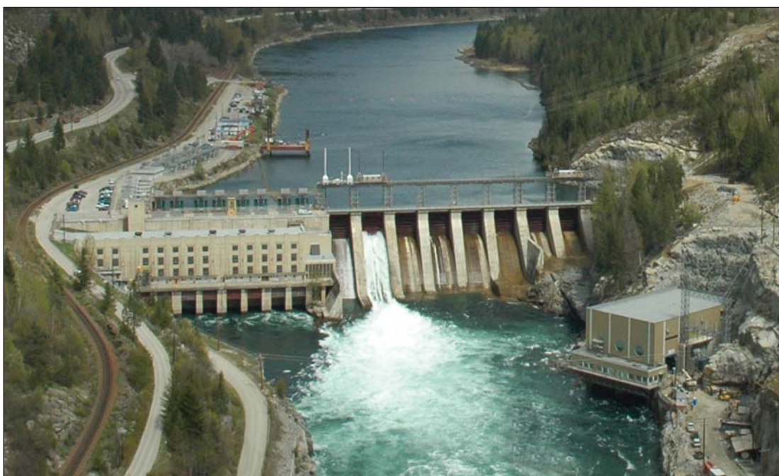
Brilliant Dam and Brilliant Expansion (under construction)
