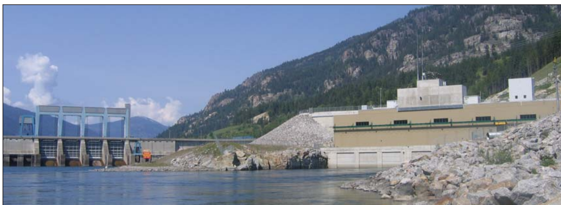
Arrow Lakes Generating Station
