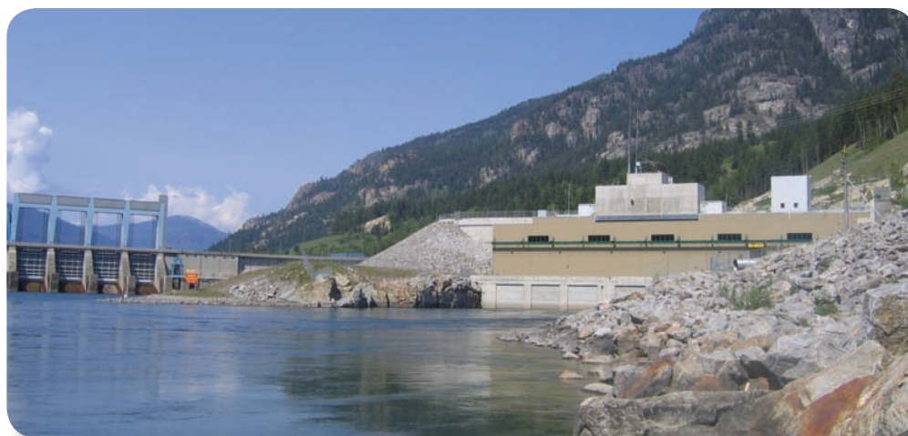
Arrow Lakes Generating Station (right) is immediately downstream of BC Hydro's Hugh Keenleyside Dam
