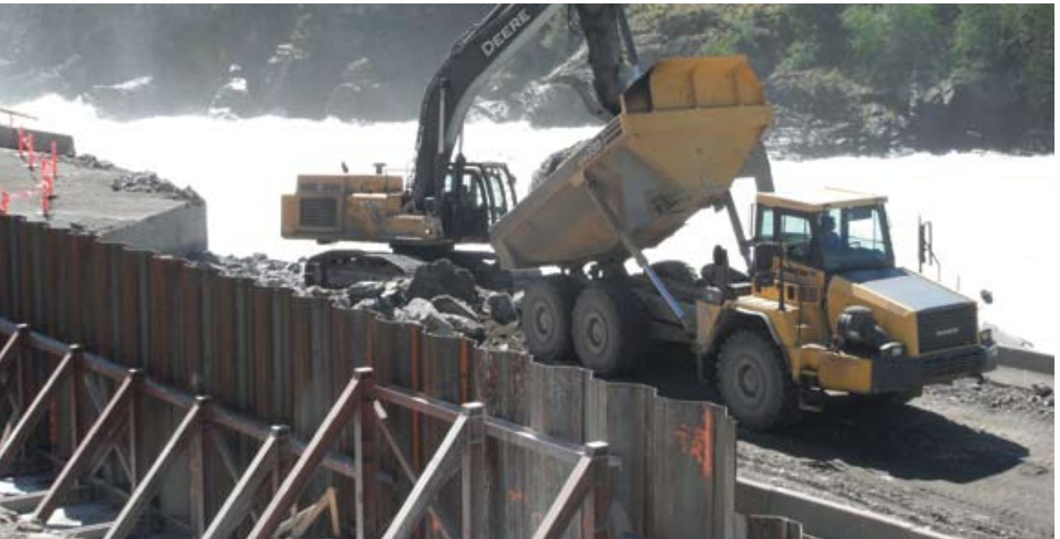
Below: Berm construction at the Waneta Expansion Project.
