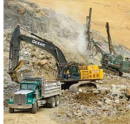
Above: Excavation of the powerhouse begins.
