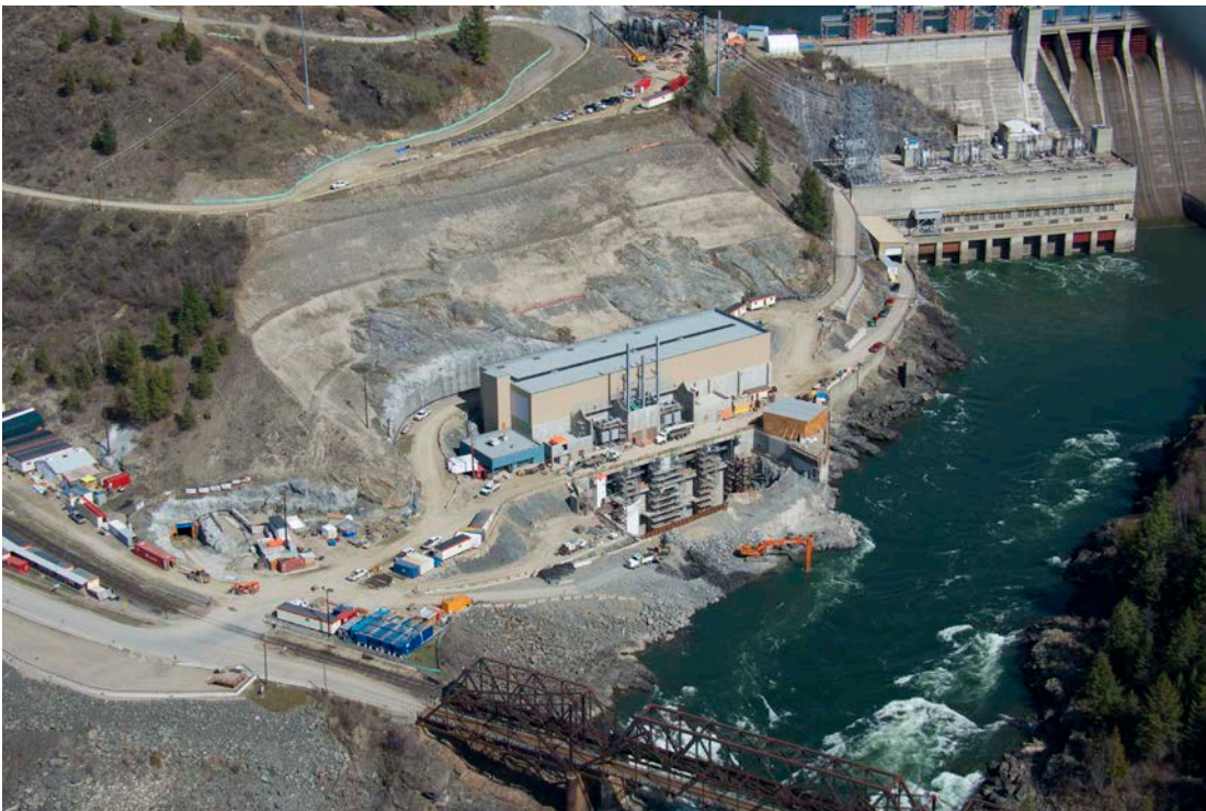
Aerial view of the Waneta Expansion Project
