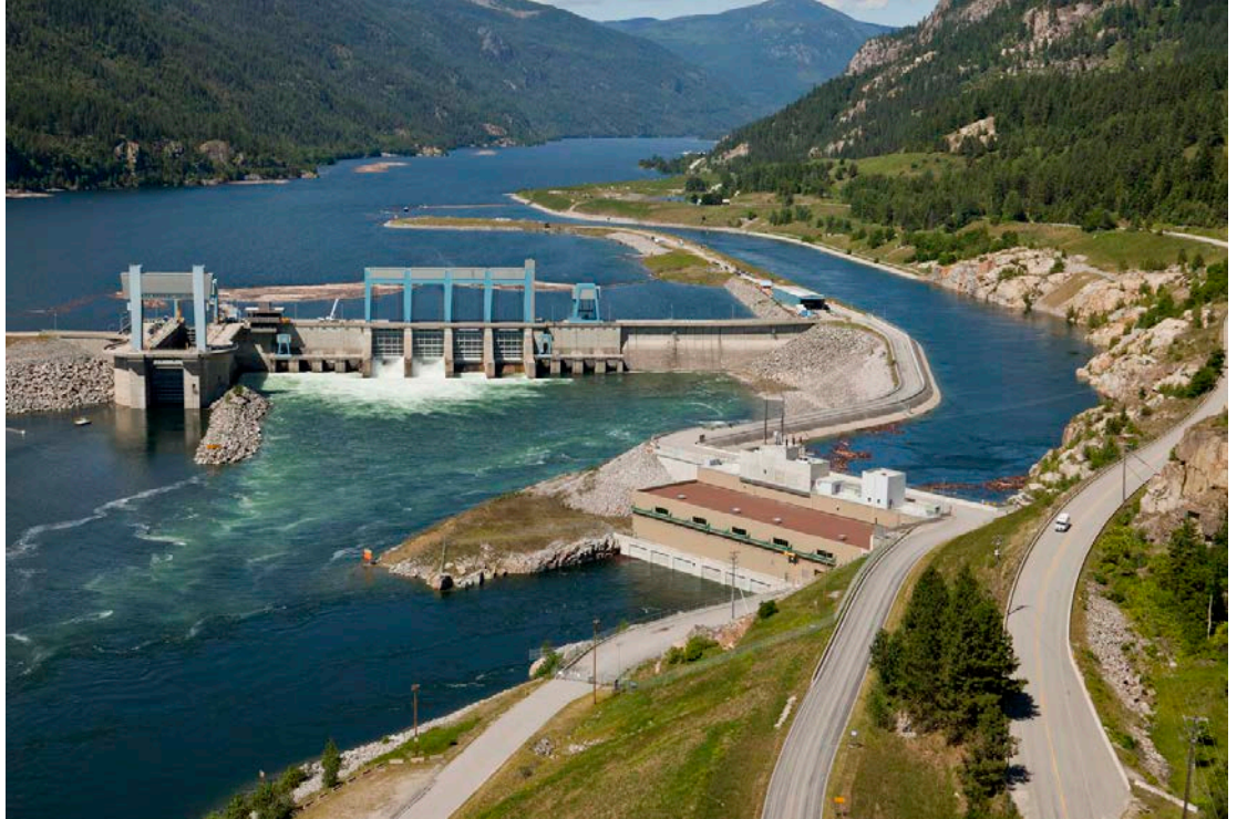
Arrow Lakes Generating Station with BC Hydro's Keenleyside dam in the background
