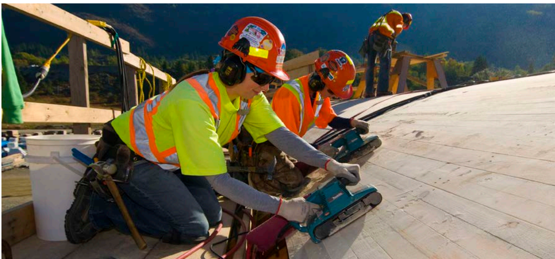
Carpenters constructing forms at the Waneta Expansion Project
