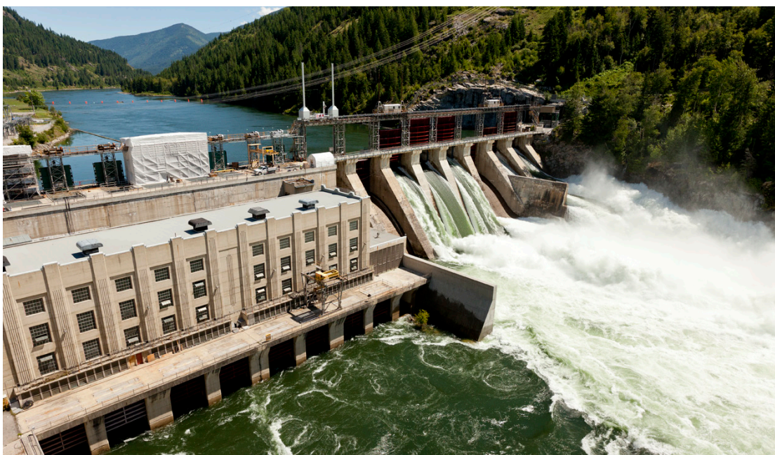
Brilliant Dam and Generating Station
