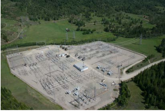
Brilliant Terminal Station
