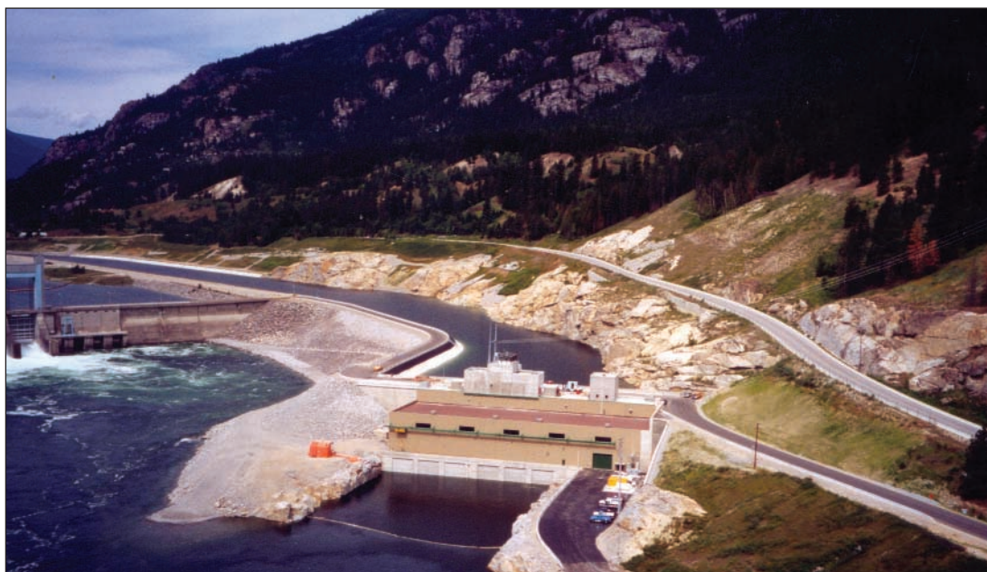
Arrow Lakes Generating Station
