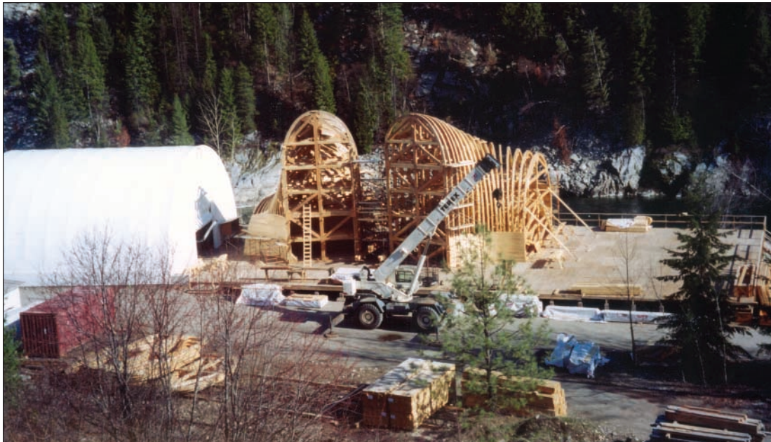
Construction of draft tube forms for the Brilliant Expansion
